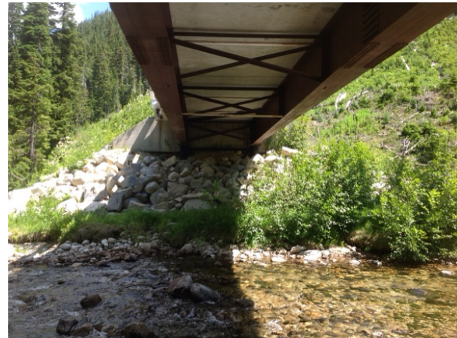
Right Bank Abutment when facing downstream
