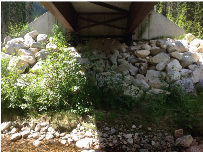
Left Bank Abutment when facing downstream
